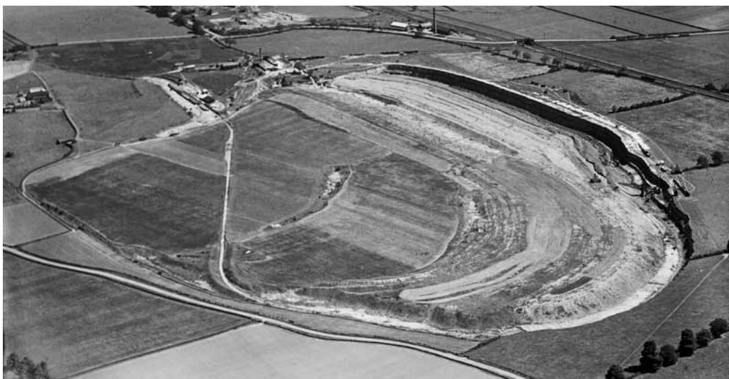
Figure 13.1 The Hawton Gypsum Quarry alongside Bowbridge Lane, Hawton in 1933. Britain from Above EPW041605. © Historic England
