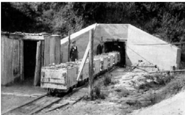
Figure 6.7 A fully laden train of clay carts exits the adit at a Dorset ball clay mine. © BCHS
