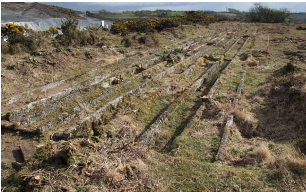
Figure 6.6 Mica drags at the Hemerdon china clay works, Devon in 2012. The site has since been completely destroyed by the advance of clay working. © Phil Newman
