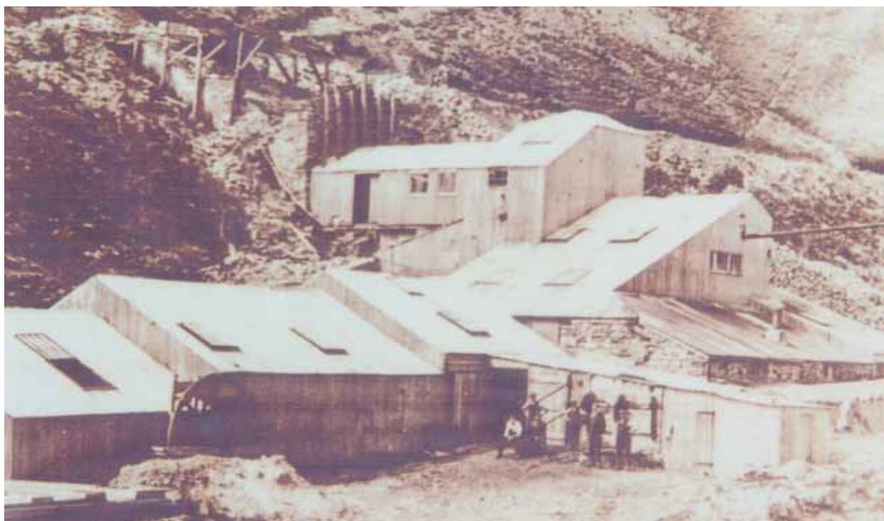
Figure 12.10 The Carrock Mine tungsten mill in operation during the First World War. © Warren Alison
