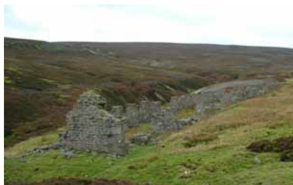
Figure 7.15 Ruins of the large peat store at Old Gang Mine in the Yorkshire Dales, showing roof support pillars and open sides. © Phil Newman
