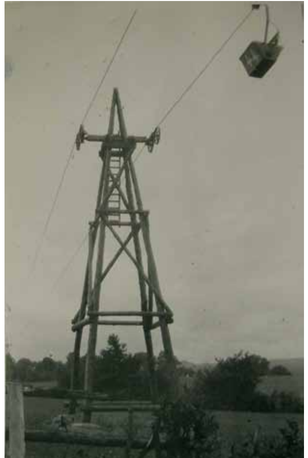
Figure 11.5 A ropeway, one of two operating between 1918 and 1948 which served Malehurst Barytes Mill, Pontesbury Shropshire, one from Bog Mine and one from Huglith mine. © SCMC
