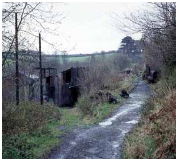
Figure 11.6 Rusting sheds and tram rails at the Bideford Black dressing sheds in 1970. © Michael Messenger
