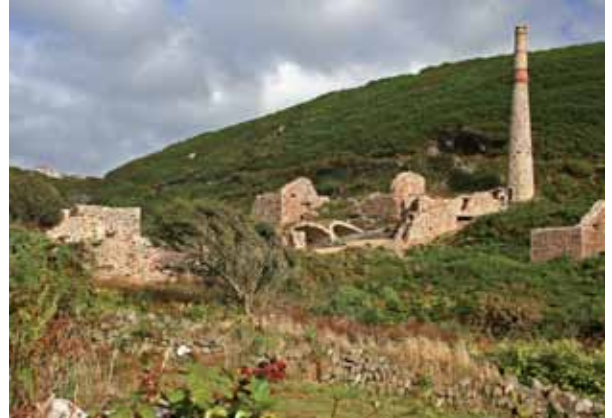
Figure 8.9 Dressing floors and calciners at Carn Praunter in the Kenidjack valley, St Just, Cornwall. © CMWHS/Barry Gamble
