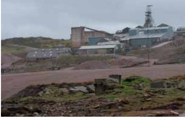
Figure 8.10 Geevor was among the last Cornish tin mines to close in 1990, but much of the surface installation has been preserved as a tourist attraction. © Phil Newman
