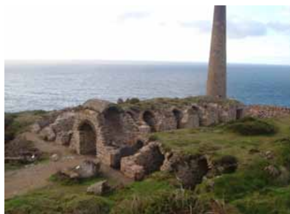
Figure 12.5 The ruined flues and chimneys at Botalack following conservation work in the 1990s. © Pete Joseph
