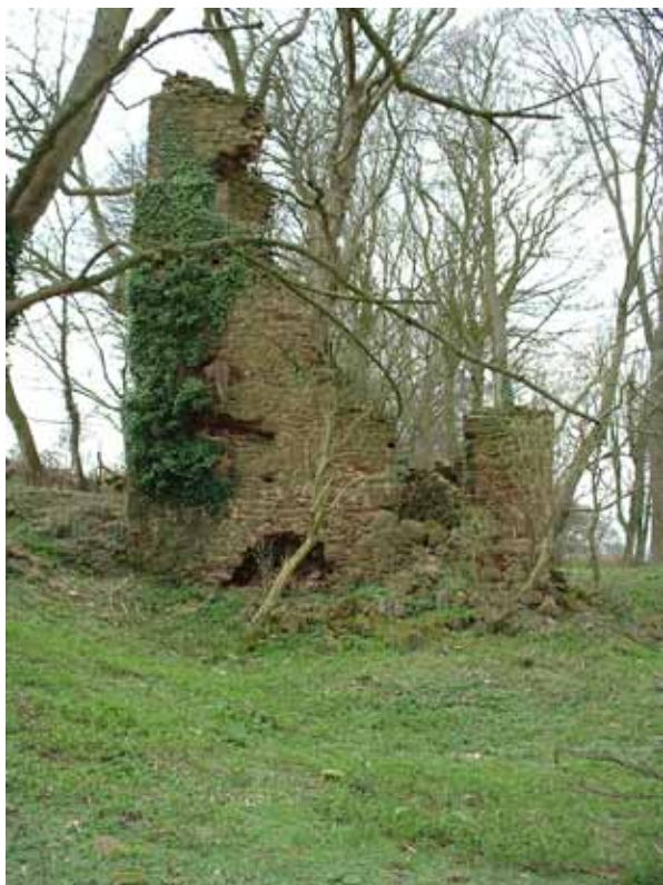
Figure 9.4 Beech Grove engine house at Doddington Mine, Somerset. Although an insignificant copper mine in terms of output, it does have two early Boulton and Watt engine houses surviving. © Phil Newman
