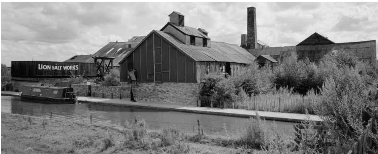
Figure 13.2 The Lion Salt Works, Cheshire viewed from the north, July 1990. Bob Skingle, © Historic England
