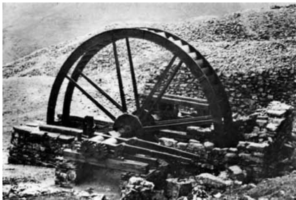
Figure 7.13 The water-powered roll crusher in situ at Old Providence, Kettlewell in the Yorkshire Dales. It was later removed and exhibited at the Dales Lead Mining Museum at Earby. © NMRS
