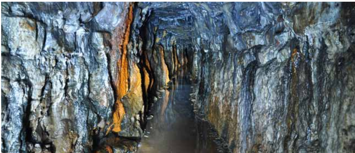
Figure 14.2 Horse haulage level in Brownley Hill Lead Mine, Nenthead, Cumbria. Probably driven before 1800. Walls coated with stalactites and secondary minerals of manganese and zinc. © James Heaton
