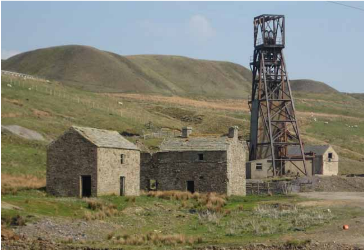
Figure 11.8 The head-frame at No2 shaft, Grove Rake - still a significant feature in the historic mining landscape in the Rookhope valley, north of Weardale. The head-frame at the adjoining No 1 shaft was stolen for scrap a few years ago. © Peter Cloughton
