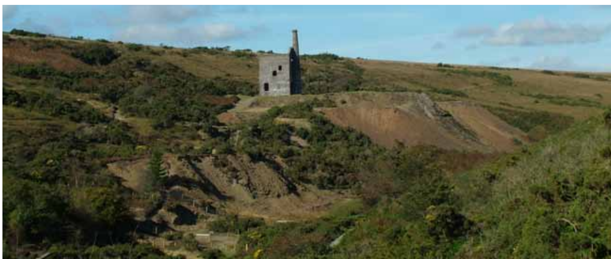
Figure 7.1 The 60-inch pumping engine house of 1868, set amid the spoil heaps at the head of Job's Shaft at Wheal Betsy is one of Devon's iconic mining structures. The mine produced lead, silver and probably some zinc. © Phil Newman
