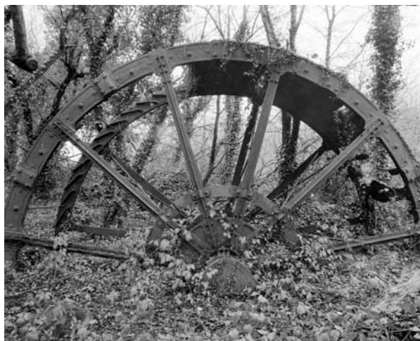
Figure 6.10 Derelict waterwheel for powering pumps in a nearby china clay pit, St Stephen in Brannel, Cornwall. Jamed Davies, © Historic England
