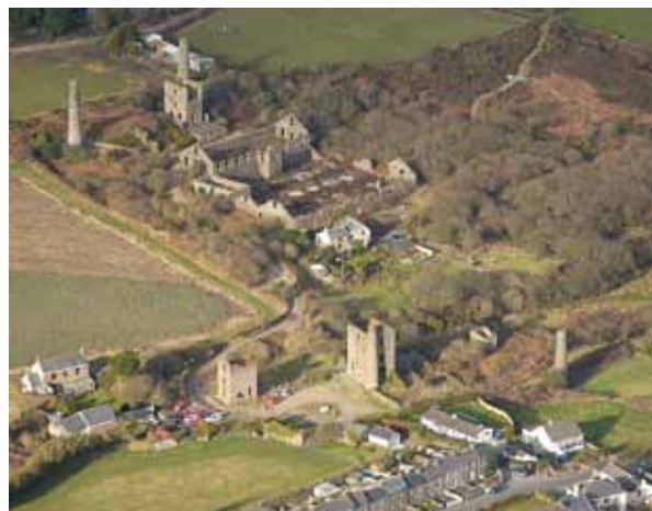
Figure 9. 8 The extensive, well-preserved and much studied surface remains of tin stamps and dressing floors at West Wheal Basset in Cornwall, date from the 1870s. However, this, together with other mines in the Camborne district had been an important producer of copper earlier in the 19th century, for which surface archaeology is less well studied. Steve Hartgroves, © Cornwall HER
