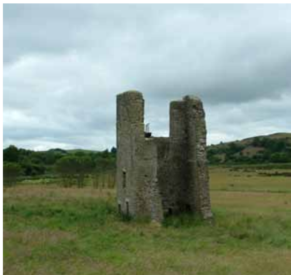
Figure 7.4 Southwest Shropshire contains a small cluster of lead mines west of the Stiperstones district. This engine house at White Grit Mine is one of several that survive in an upstanding state. © Phil Newman
