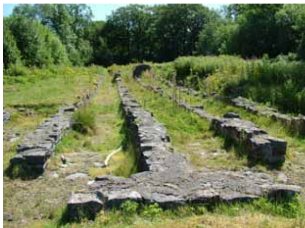
Figure 7.16 Remains of the flues attached to the lead smelter at Charterhouse on Mendip in Somerset. © Phil Newman
