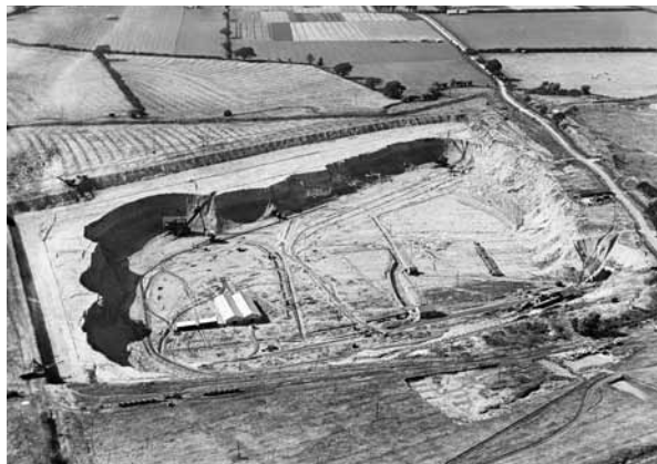
Figure 6.5 Oxford Clay extraction at the Pillinge Brickworks, Beds 1930. © Britain from above EPW033897
