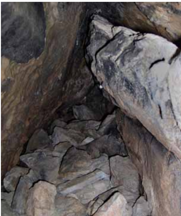
Figure 15.1 Evidence of firesetting at Old Hen Mine, Hassop, Derbyshire. Potentially dateable charcoal may be found in the debris at the base of the fired area. © Adam Russell
