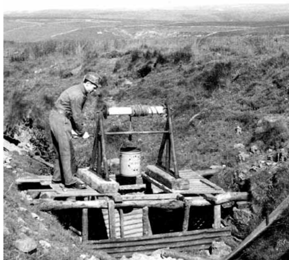
Figure 7.9 The windlass or jackroll was a common method of hauling in shallow lead works, used at surface and below ground over many centuries. © NMRS
