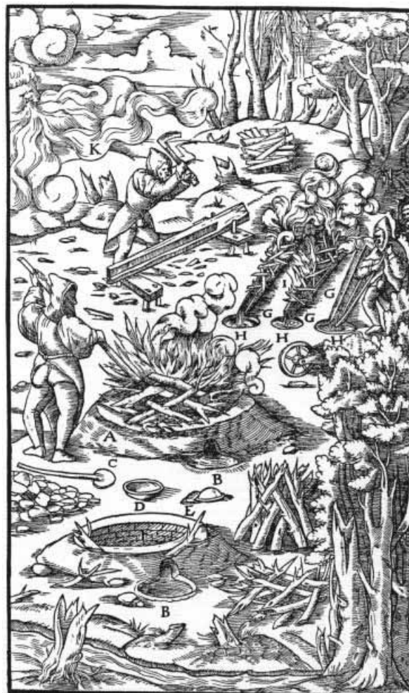
A—PIT ACROSS WHICH WOOD IS PLACED. B—FOREHEARTH. C—LADLE. D—IRON MOULD. E—CAKES. F—EMPTY POT LINED WITH STONES IN LAYERS. G—TROUGH. H—PITS DUG AT THE FOOT OF THE TROUGH. I—SMALL WOOD LAID OVER THE TROUGH. K—WIND.
