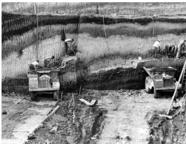
Figure 6.3 Ball clay being cut by 'spaders' in a Bovey Basin clay pit during the 1950s. Note the varied stratigraphy of the deposits. © BCHS
