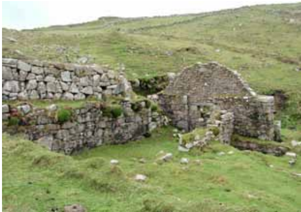
Figure 8.8 Castle Stamps, Porthmoina, West Penwith. Remaining structures of a water-powered stamping mill of the earlier 19th century. The curved-top wall is the splash wall on the west side of the wheelpit. The axle from the wheel to the stamps passed through the squared opening. © Phil Newman
