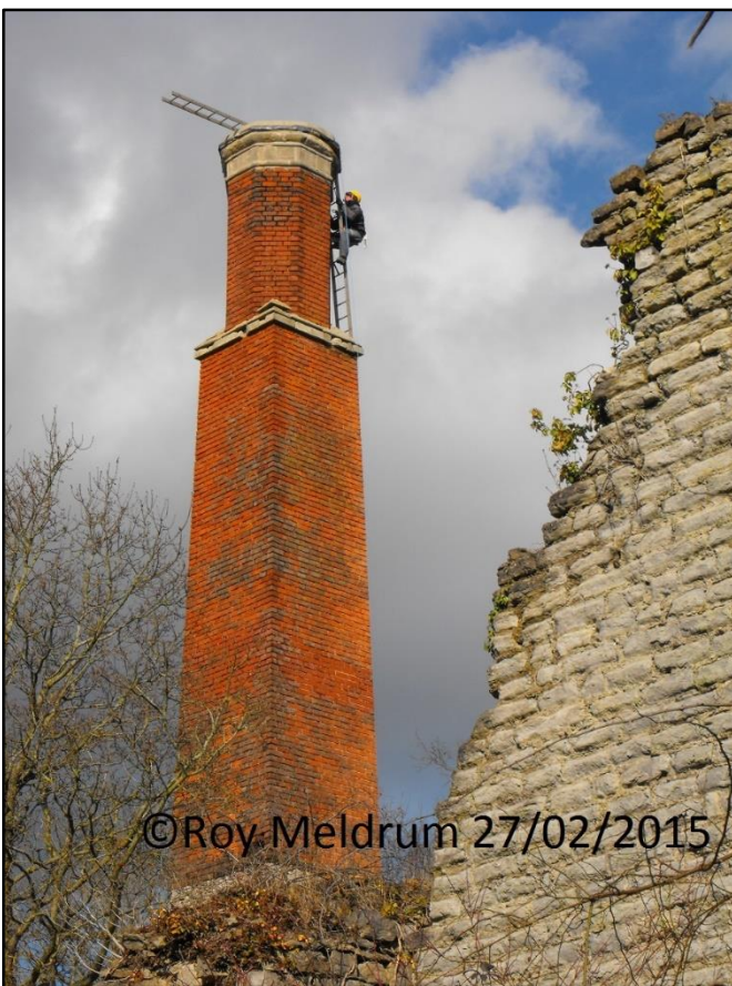
Repair work underway, Brandy Bottom Colliery
