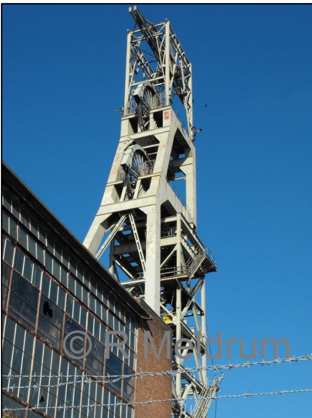
Clipstone Colliery downcast headstocks 2010
