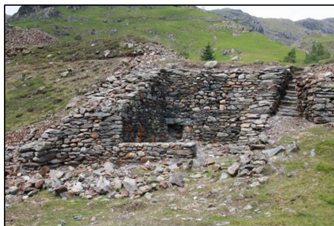
The same building at Low Bonsor Mill after consolidation
