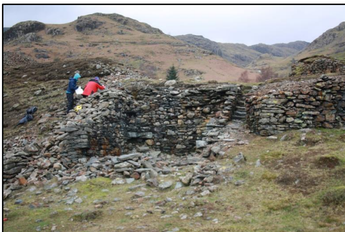
One of the buildings at Low Bonsor Mill before restoration
