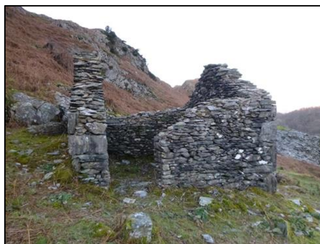
The powder house has been partially rebuilt
