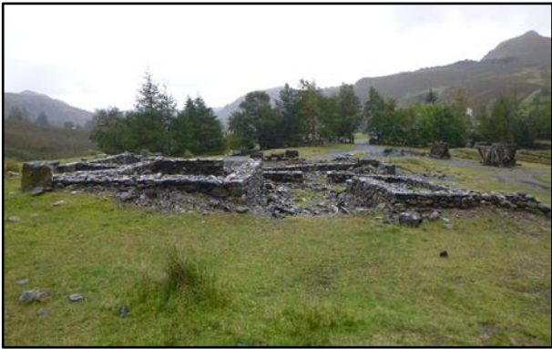
Walls of the smithy have been consolidated
